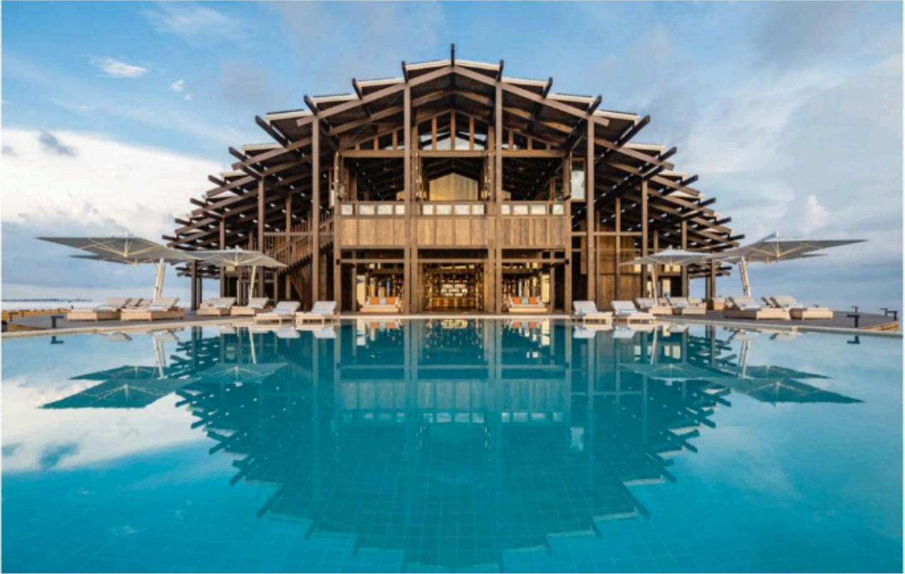
Above: The roof of The Retreat is clad in 984 solar panels collectively generating enough energy to power the entire resort
